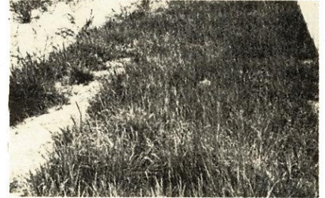
A vegetative filter strip keeps sediment off the road in a new subdivision.
