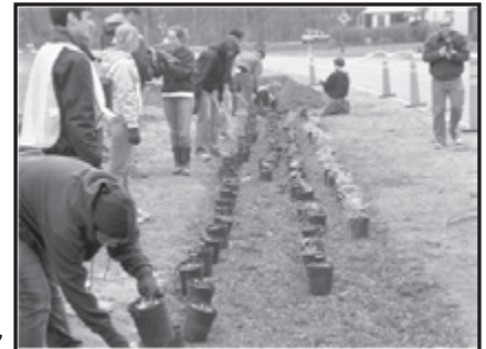
Notre Dame Students Installing Rain Garden. Image Source: CARDNO JFNew’s website at www.cardnojfnew.com
