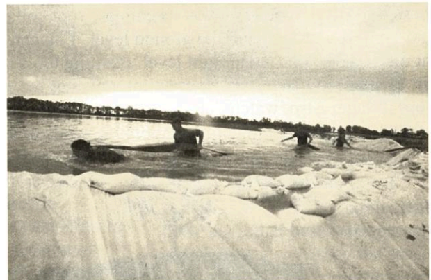
Marines and sailors move a hose through water from the White River in Elnora, Indiana on June 9, 2008 to help state and local authorities raise the White River levee in an attempt to prevent further flooding in the area. (U. S. Marine Corps photo by Lance Cpl. Patrick M. Johnson-Campbell.)
