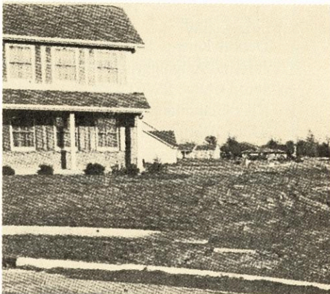
Use of dormant seedling could have reduced excessive early spring erosion on this site.
