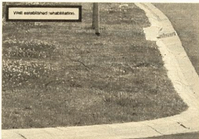
This filter strip along the road is helping protect the storm drain from receiving sediment and other pollutants through surface runoff.
