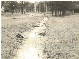
Water collects in a roadside swale, resulting in filtration of pollutants from the water.
