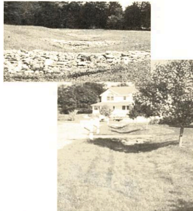
Top: A grassy swale with rock check dams slows runoff velocity. Bottom: A turf grass lined swale improves stormwater quality in a subdivision.
