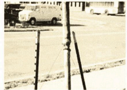
Tree stakes can be very helpful but you need to remove them before they interfere with the tree's growth. Here the cables are girdling the tree and the top is larger than the bottom.
